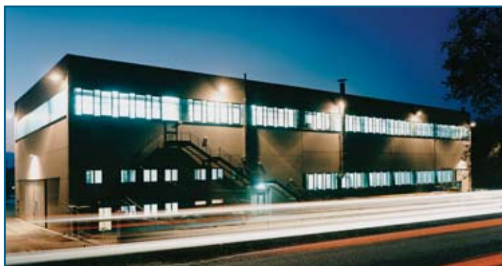
Sede Produttiva pistoni - Monvalle (Italy) Piston manufacturing plant - Monvalle (Italy)
